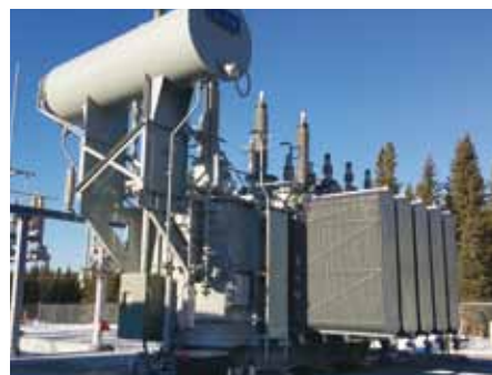
CANADA, 3 PHASE 138kV 42MVA
